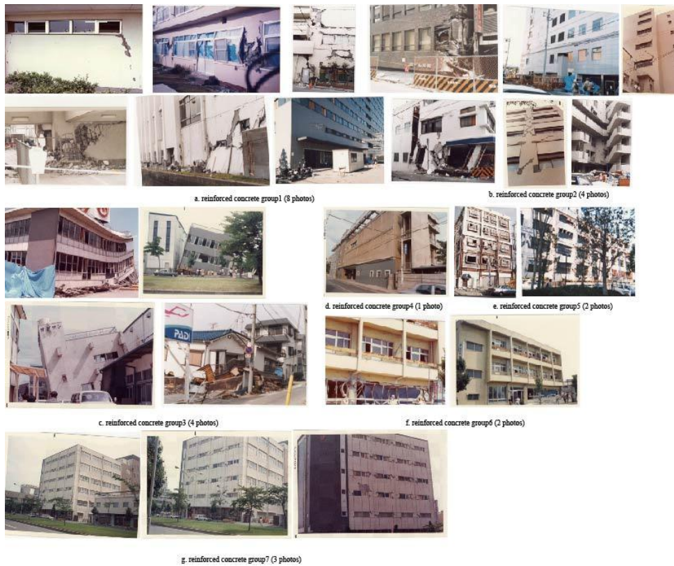
Fig.2 Damaged photographs of frame structure
