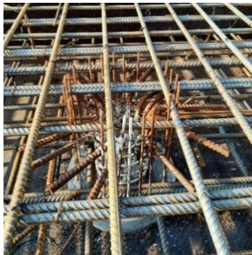
Figure 1. Spun pile-to-pile cap connection
