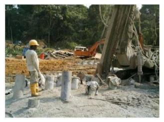
Figure 10. Slightly inclined micro- piles [6]
