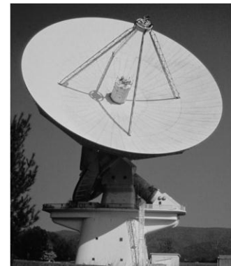
Figure 1. schematic of the national radio astronomy observatory (NRAO) telescope, located in West Virginia, USA. The reflectors are made from aluminum
