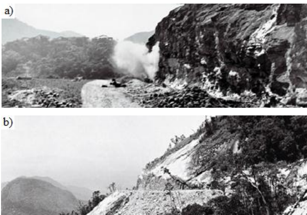
Figure 4. Construction of the Rio-Teresópolis highway. a) Km 25 (1968) b) Km 88 (1968) [9].
