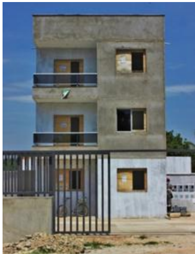
Figure 1. Front of the building (Source: Author, October/2015)
