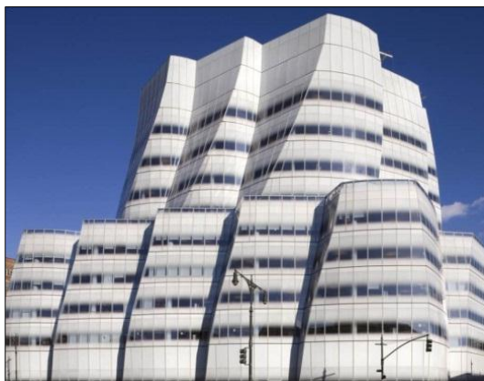
Figure 1. IAC Building in New York City, New York, USA
