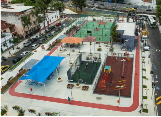
Figure 13. Praça Niterói on a detention basin with capacity for 58 million liters of water.
