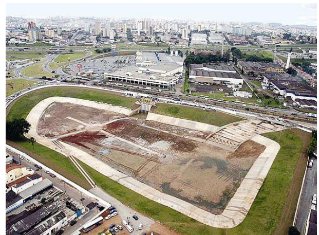
Figure 1. Detention basin of Vila Paulicea, São Paulo.
