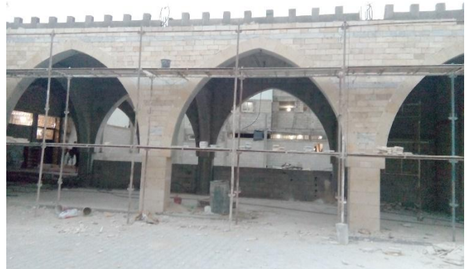
Figure 11. Al-Kozomiry Mosque their facades, they have been reconstruction from modern technology materials and cladding with ancient marble
