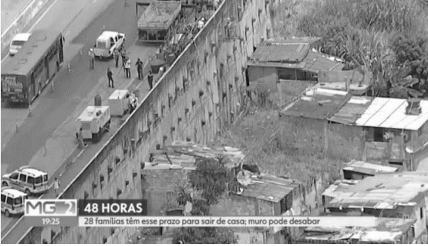
Figure 4. Houses in the immediate vicinity of the wired wall.
