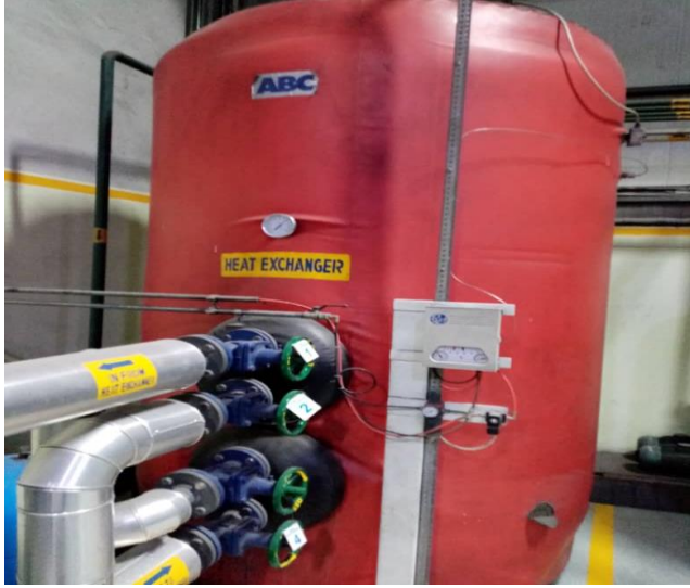
Figure 1. ABC shell and tube heat exchanger (Olam)
