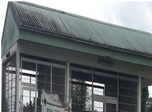
Figure 1. Gas Station roof in Uyo (Site 1)
